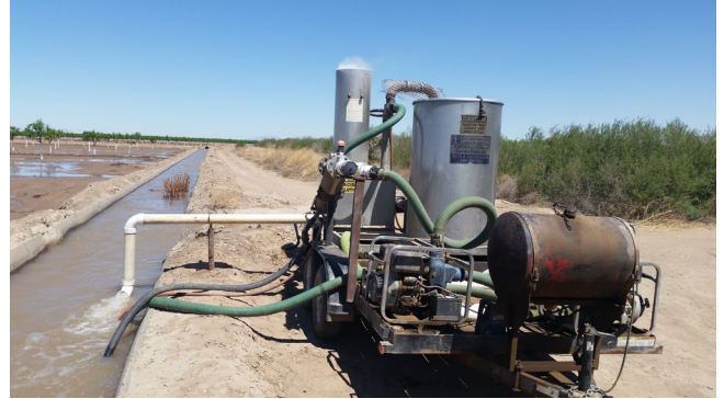
Sulfur burner is treating irrigation water in the field
