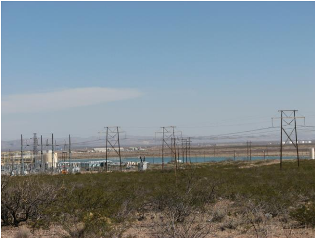
Cooling Tower Reject Water stored in a pond at El Paso Electric Newman power plant in northeast El Paso, TX.
