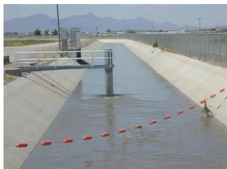
Lined American Canal Extension in El Paso
